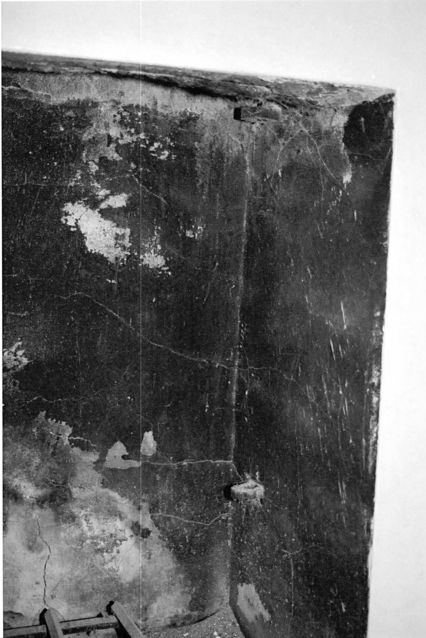
Photo 13 of 18: East chamber fireplace, south jamb with crane eyes. 11/5/2019
