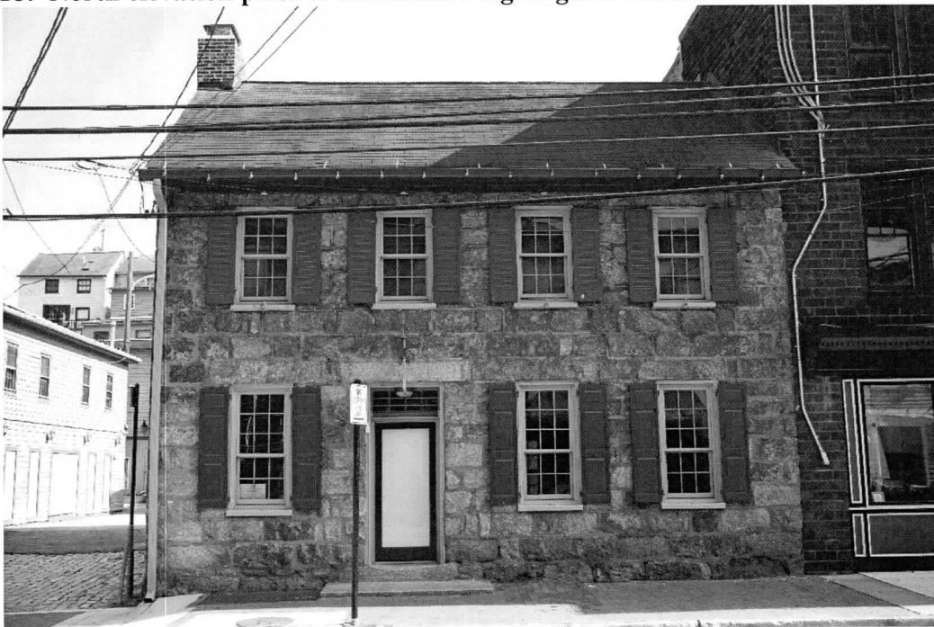
Photo 2 of 18: North elevation after floods showing replacement windows and shutters. 8/25/2020
