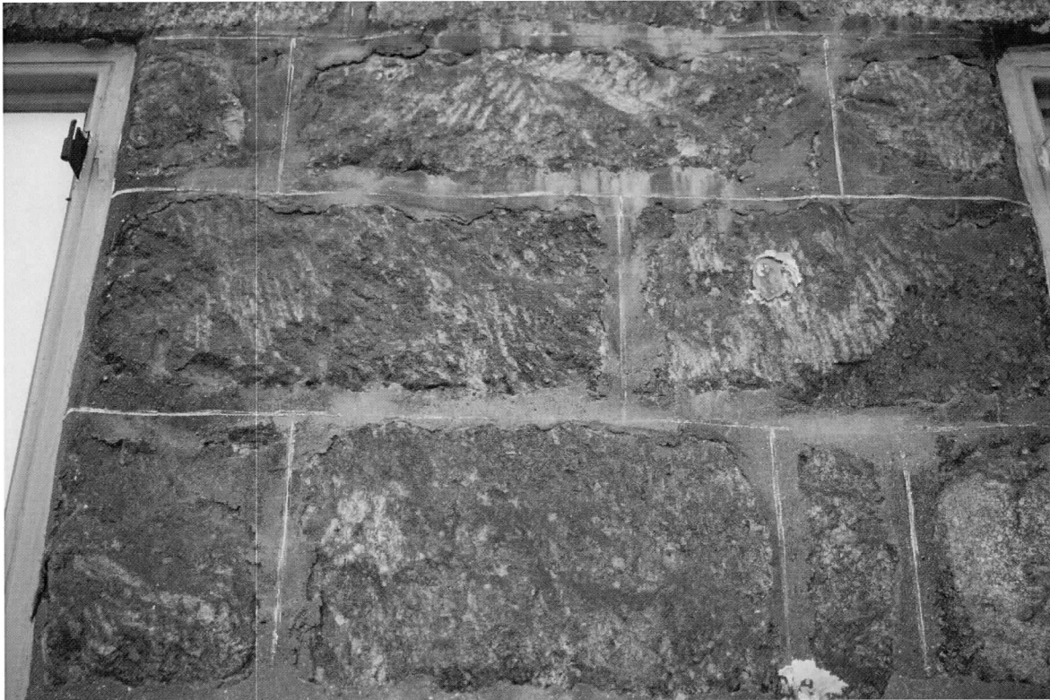
Photo 3 of 18: North elevation pencilling. 3/27/2019
