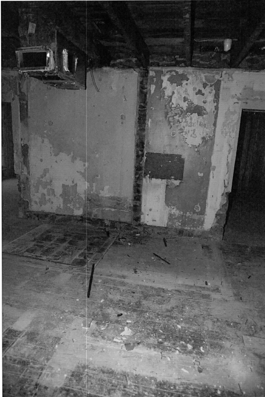
Photo 15 of 18: Second story, view south showing ghosts of missing partition walls on floor and wall following removal of later material. 11/20/2019
