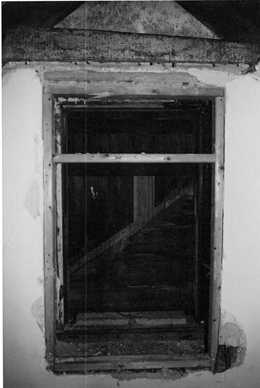
Photo 16 of 18: Attic, west window. 11/5/2019
