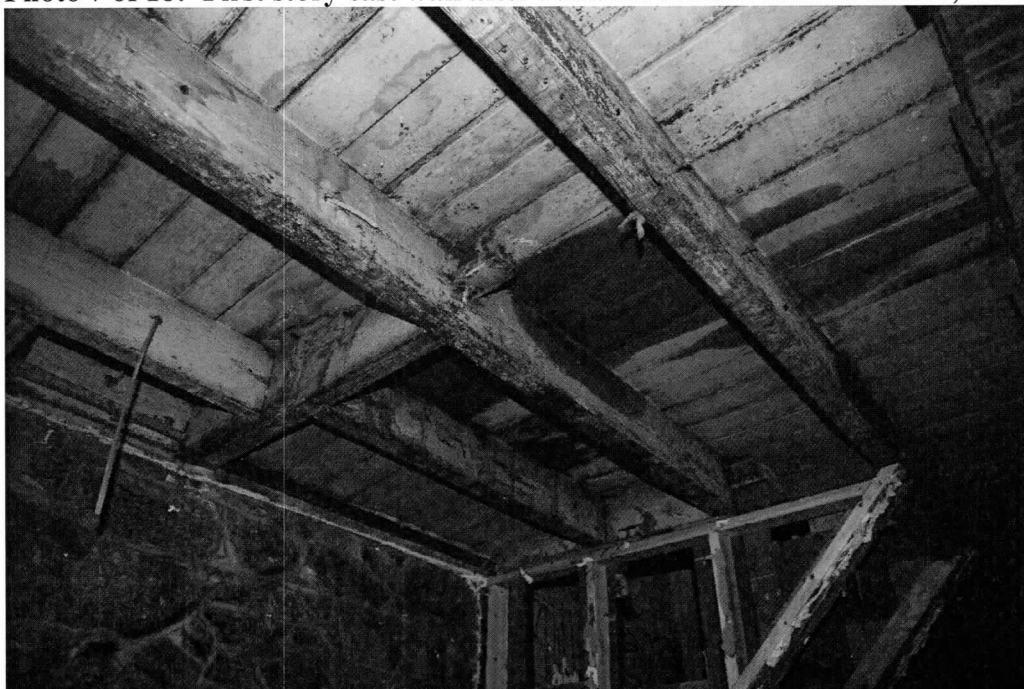
Photo 8 of 18: First story ceiling framing at east end. 11/5/2019
